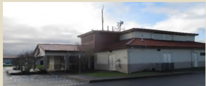
Emergency Operations Center, Building 7022
