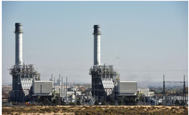
The Hermiston Generating Plant provides power for nearly 500,000 households in the Pacific NW, courtesy of Perennial Power.
