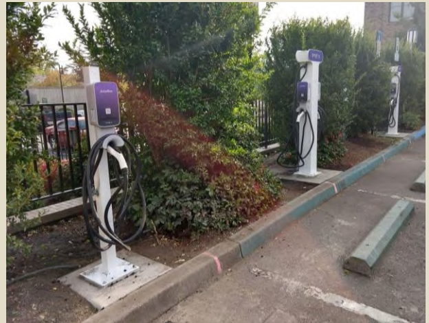
In 2020, the City of Ashland installed free public EV chargers using Oregon Clean Fuels Program credits.
